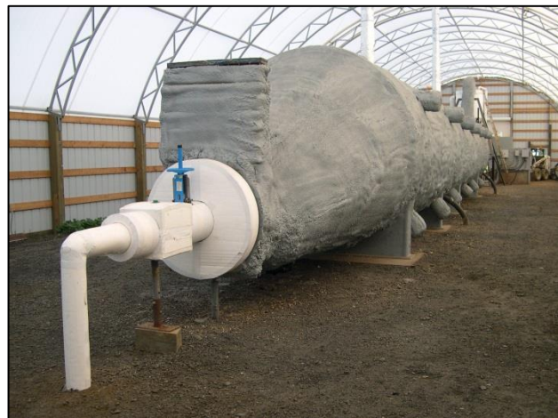
Figure 1. Avatar AnD 1B22 digester at Keewaydin Farm. Photo courtesy of Charles Gould.
