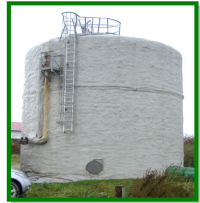
Nordic Farm's experimental digester
